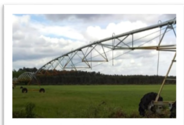
Irrigation (Source : SBHG)
